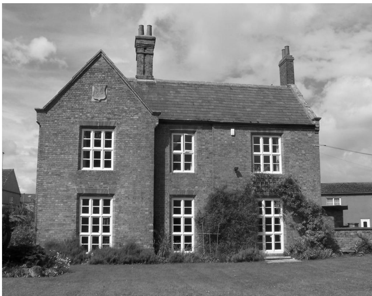
Billingborough Vicarage - the architect was Thomas Pilkington, who also did alterations to the fine parsonage at Market Deeping.
